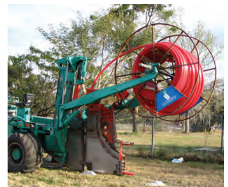
Plow chute installation
